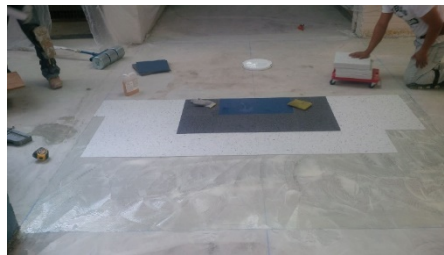
After CSP – 1 w/ Aquaflex Waterproof Patch
