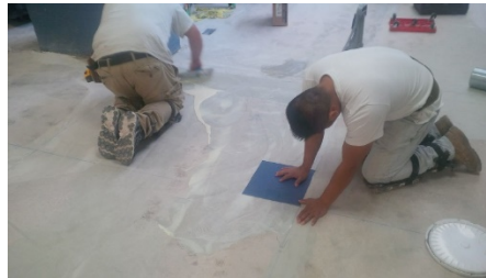
Troweling Aquaflex | Starting Point in Corridor Intersection
