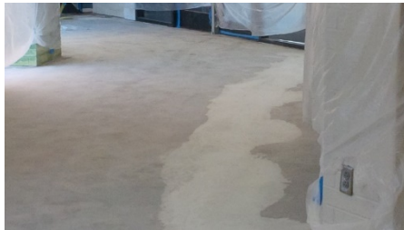
After CSP – 1 w/ Aquaflex Waterproof Patch
